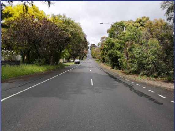
Figure 7: Manchester Road (eastern carriageway) – view south
