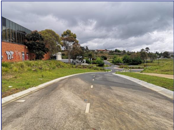
Figure 8: East Ridge Drive – view north-west
