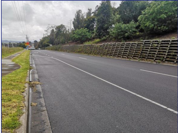
Figure 6: Manchester Road (western carriageway) – view north
